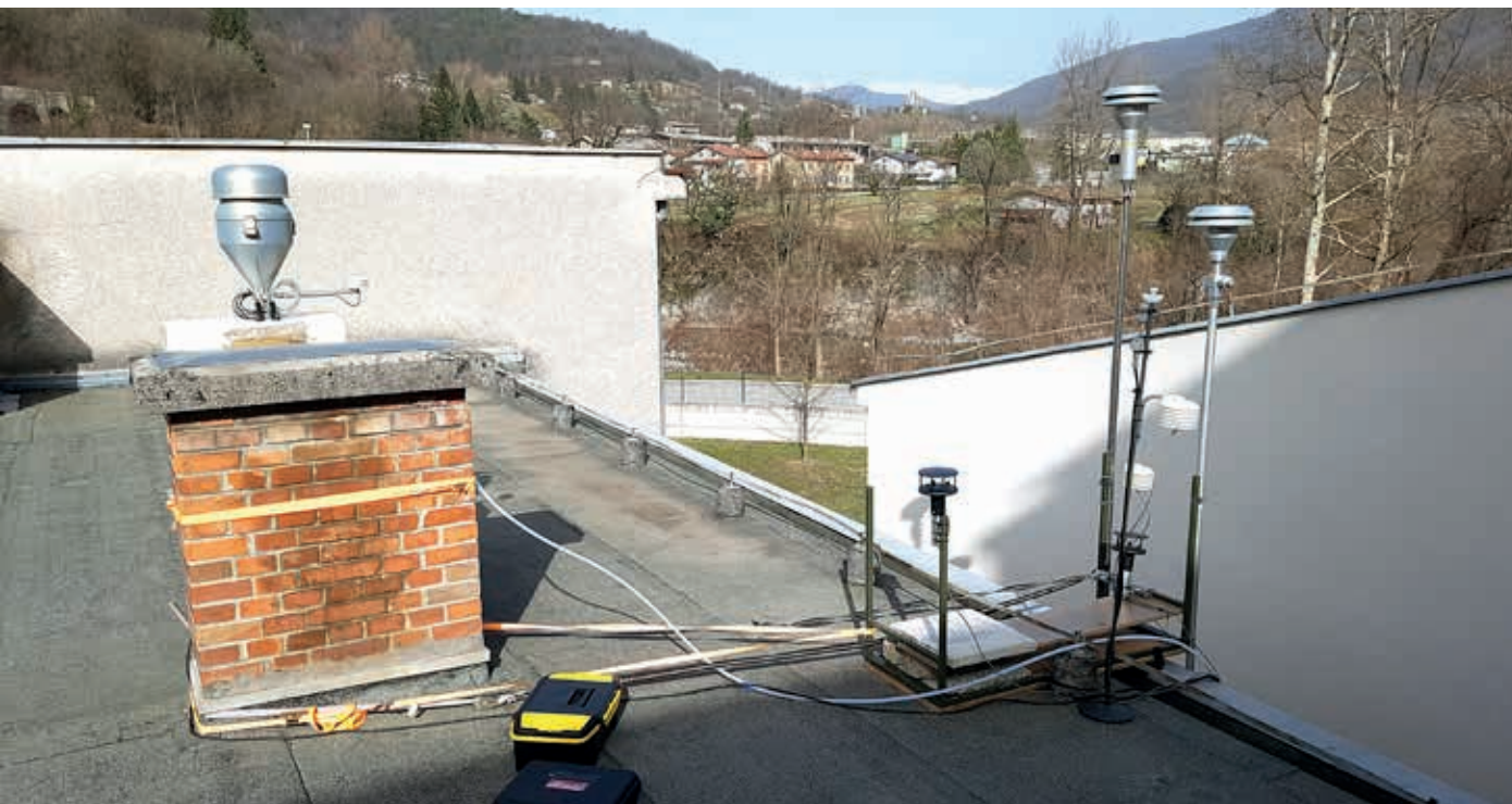
Sampler and Inlets for air quality measurements in Kanal ob Soči municipality.
